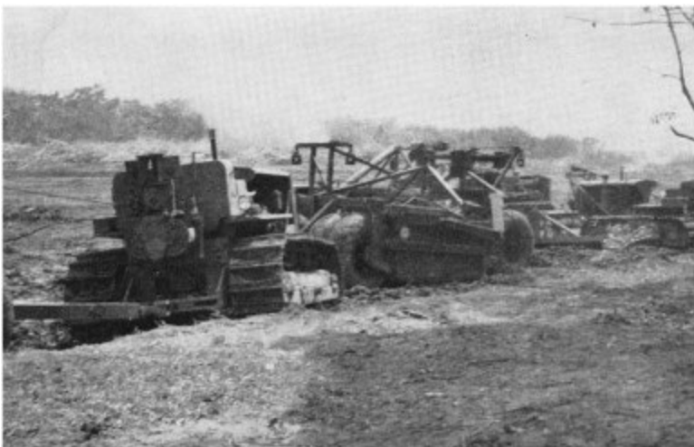
No. 1 Aerodrome Construction Squadron preparing the bomber strip at Tebrau, Malaya
