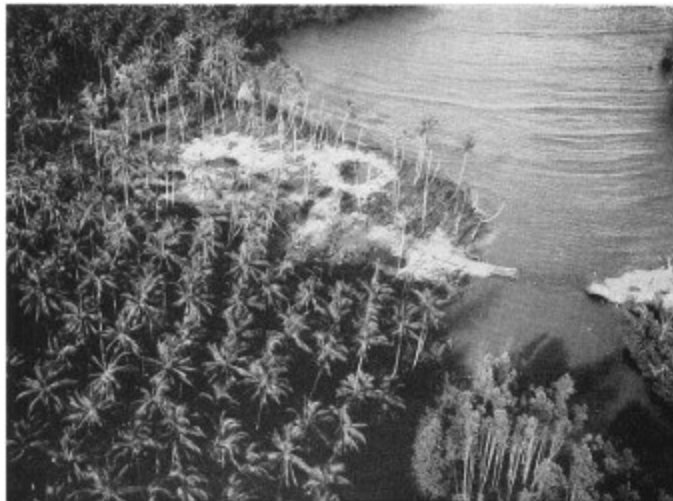
Bridge on the East Coast of New Ireland, February 1944, after low-level bomb attack
