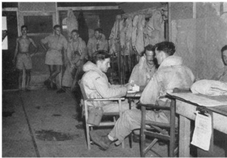
Corsair pilots in crew room, Bougainville, January 1945
