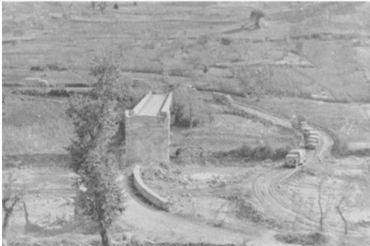
A bridge near Gissi, demolished by the retreating enemy, and alongside it the deviation made by the New Zealand Engineers
