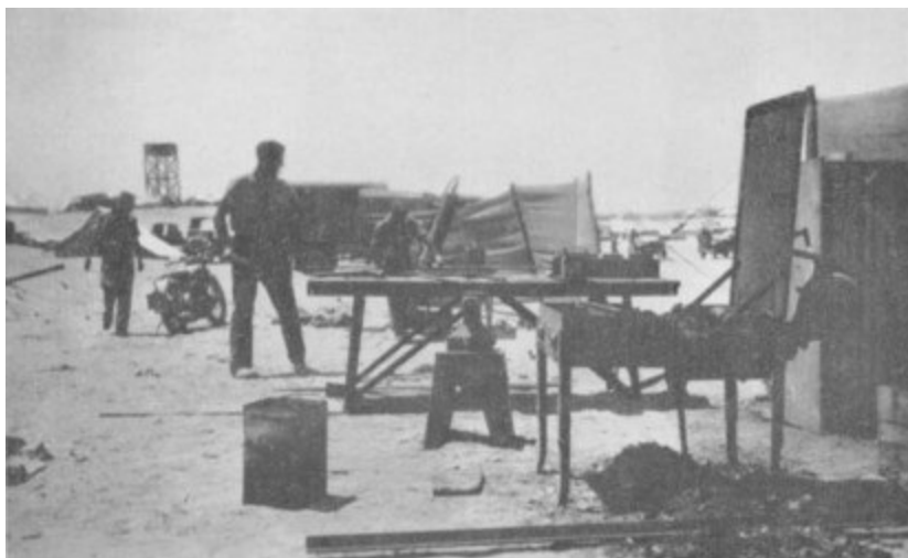
Workshops Section—blacksmiths' shop, Helwan, 1941
