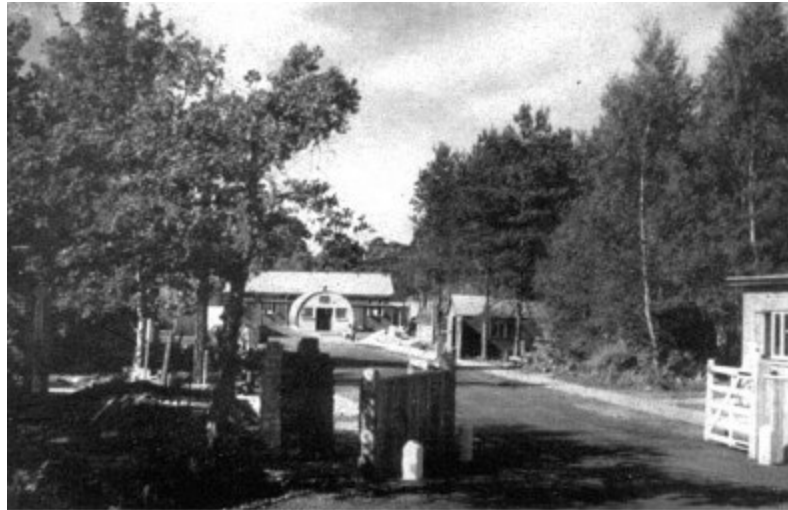
1 NZ General Hospital entrance, Pinewood, England
