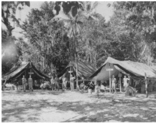
Indian pattern tents, raised high on poles to give added ventilation and headroom, form the wards of the 22 Field Ambulance hospital near Tanaheran, Nissan
