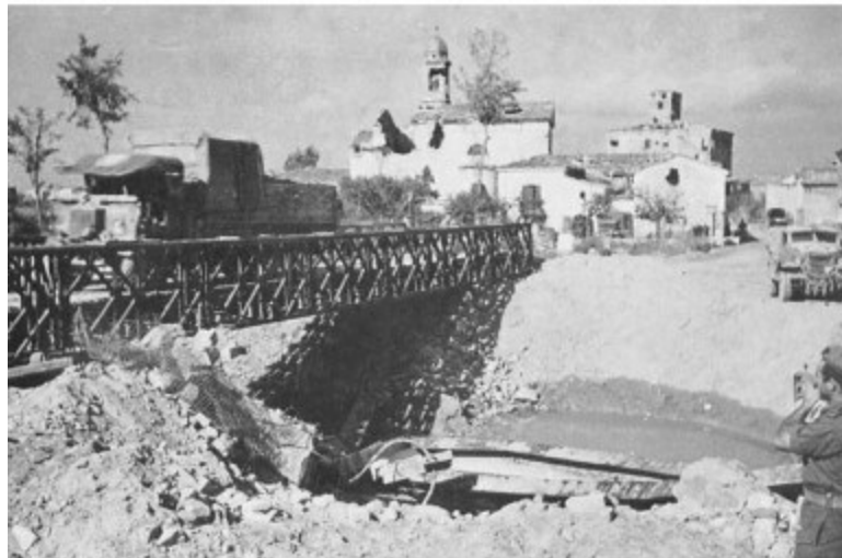
The Bailey bridge over the Scolo Rigossa on the way into Gambettola
