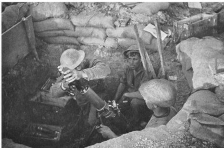
A mortar crew in action close to the Senio stopbank
