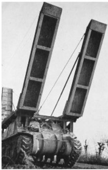
An Ark (a tank with ramps for bridging canals and ditches) on Route 9 between Forli and Faenza
