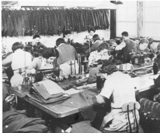
Battledress being manufactured at Cathie & Sons Ltd.
