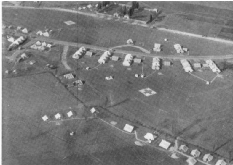
AN AERIAL VIEW OF 1 NZ MOBILE CCS on a bypass of the main road, near Cassino . The theatres and administration tents are on the left by the road, and the wards on the right
