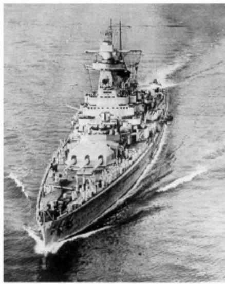
ADMIRAL GRAF SPEE mounted six 11-inch guns in two triple turrets
