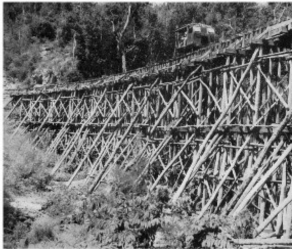
THE HINTOKU-TAMPI RAILWAY BRIDGE. Rough scrub timber has been used in the construction of this bridge, whose height was 100 feet. Note the small diesel-driven trolley. The photograph was taken in October 1945.
