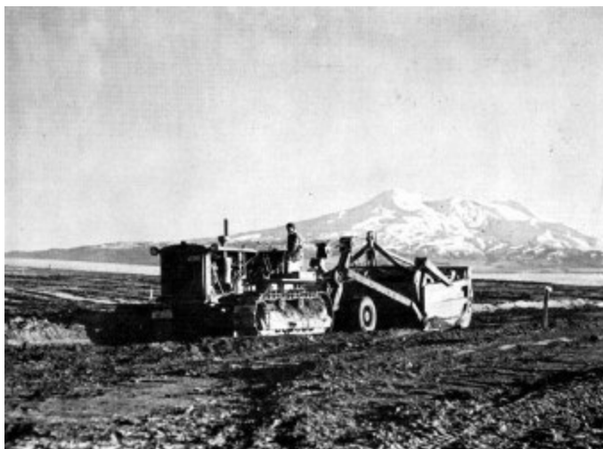
DEFENCE CONSTRUCTION Levelling the site at Waiouru Camp in August 1940
