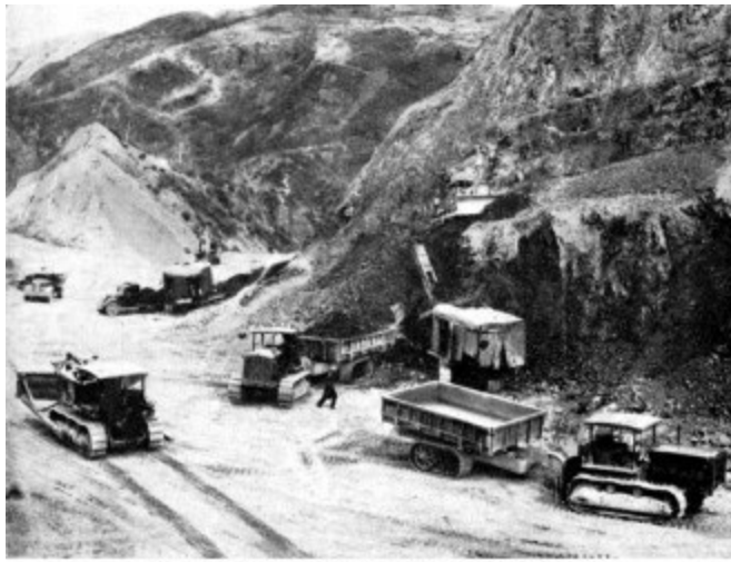
HEAVY EARTHMOVING EQUIPMENT, PRE-WAR Construction of the Ngahauranga Gorge road in 1938-39
