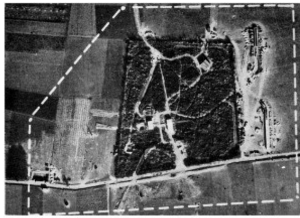
One of the first flying-bomb installations found by the Royal Air Force in Northern France. A reconnaissance photograph before the attack ( above ) and after the target had been bombed ( below )
