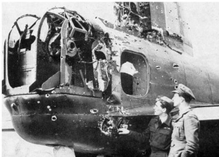
The damaged tail unit of a No. 75 Squadron Stirling
