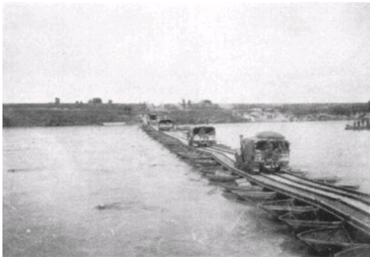
By pontoon bridge over the Adige By pontoon bridge over the Adige
