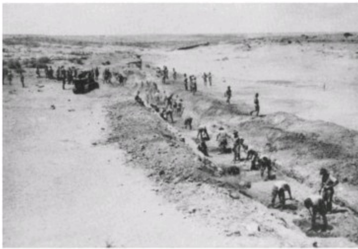
Work on a tank obstacle in Wadi Naghamish, June 1940
